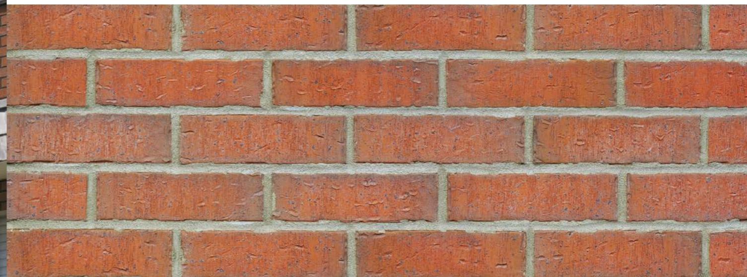
Brick tower HF03
